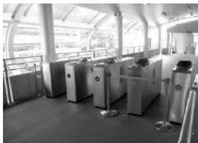
Ticketing turnstiles at entry exit to a prepaid platform area (Bangkok BRT)
