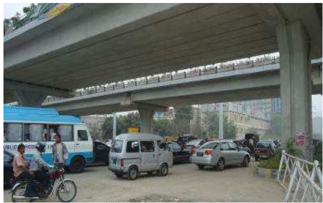
Figure 3.4.17 Kalma Chowk Flyover and Turning Traffic Below
