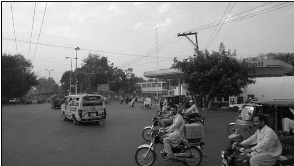
Figure 8.5.3 Poor Gyratory System Design without Traffic Channelization
