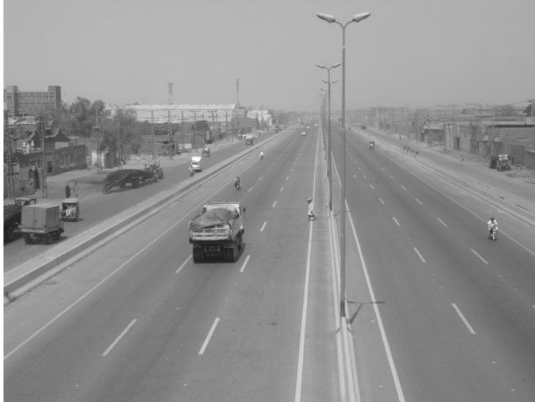
Figure 2.1.7 A Completed Section of Lahore Ring Road
